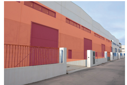
Wall protection (outdoor) at Warehouse
